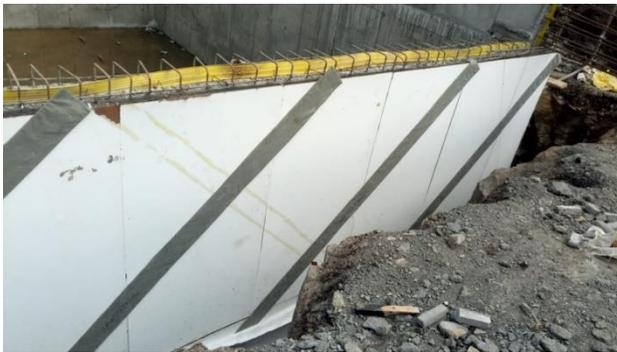
*Wickdrains<sup>®</sup> installed at 45° angle
