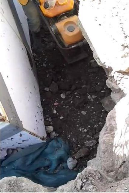
*150mm layer of murrum compacted to engineer's specification
