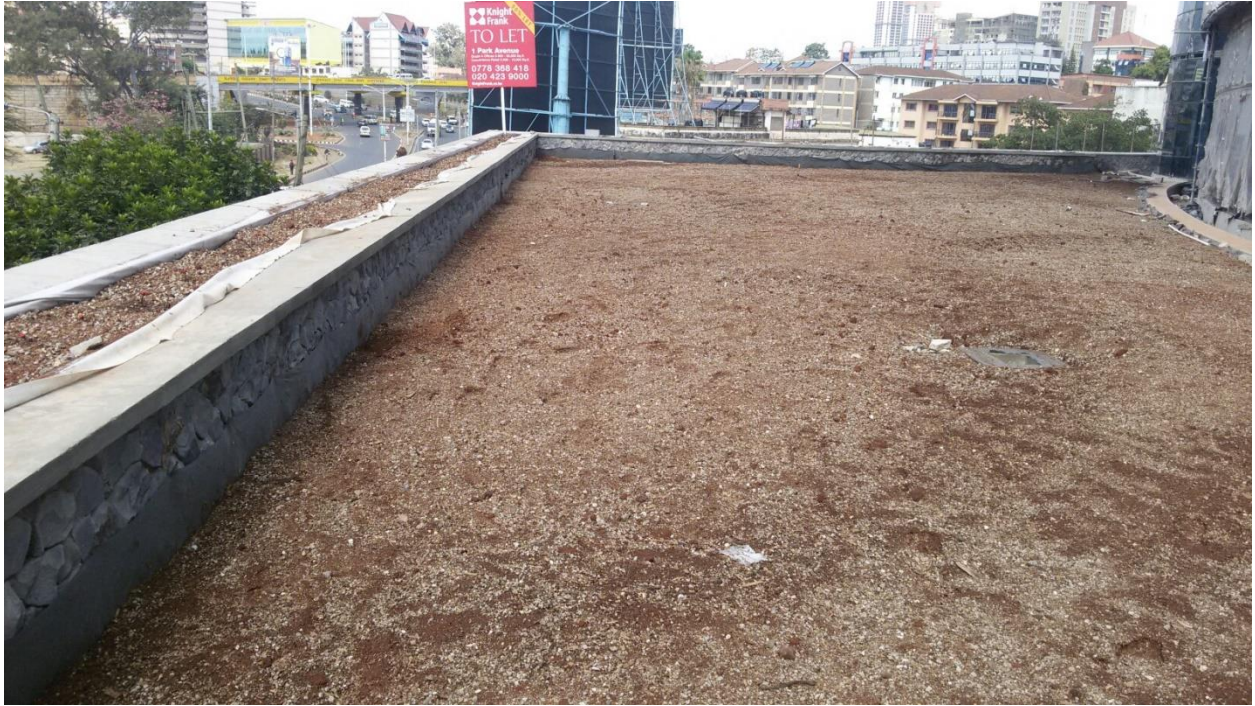
Image 3 – Top soil placed over the 150 gsm geotextile.
