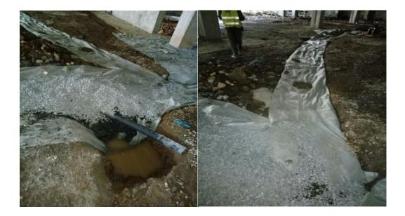
Traditionally, heavy duty UPVC pipes with slottings were used for subsoil drainage.
