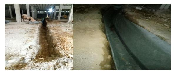
Coarse aggregate was filled at the base and the perforated HDPE pipes were laid.
