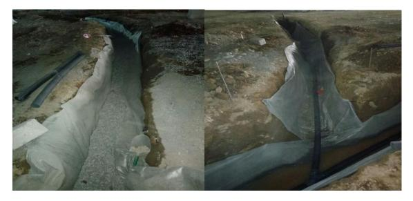
The perforated HDPE pipes were then covered with another layer of coarse aggregate and the whole was then wrapped by the geotextile material with a 300mm overlap on top.
