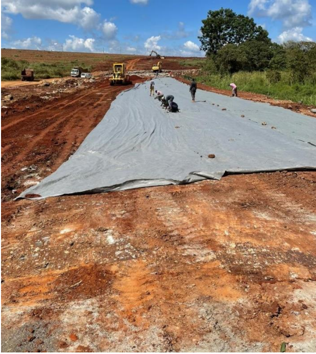
Laying the 180 gsm non-woven, needle-punched geotextile over the compacted boulders.
